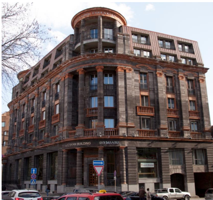
Figure 2. View of the 7-story base isolated “Tufenkian” building with non-symmetric plan of the multifunctional hotel/commercial center complex constructed in Yerevan
